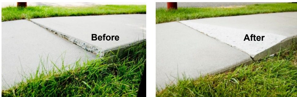
Figure 10: Precision Sidewalk Safety Work Example
