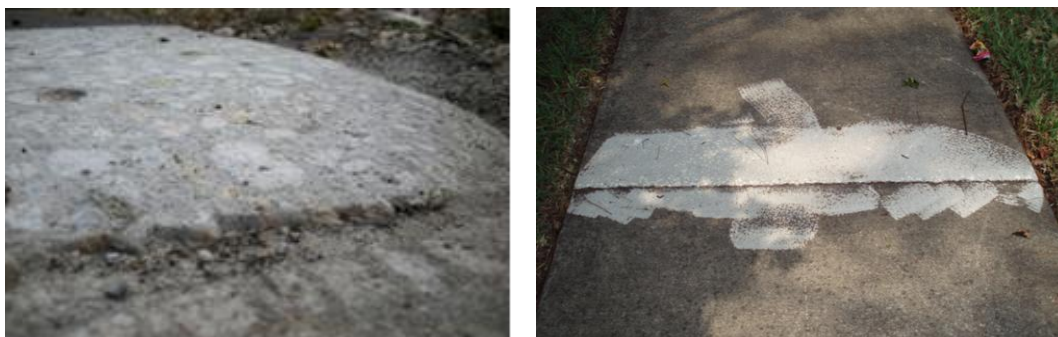
Figure 10: Typical Results from a Grinder
